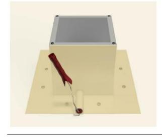
Step 11: Apply a generous amount of heat & pressure to TPO boot to weld it on to the curb & the deck.
